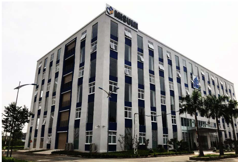
Exterior of the warehouse and office in Ho Chi Minh, Vietnam
